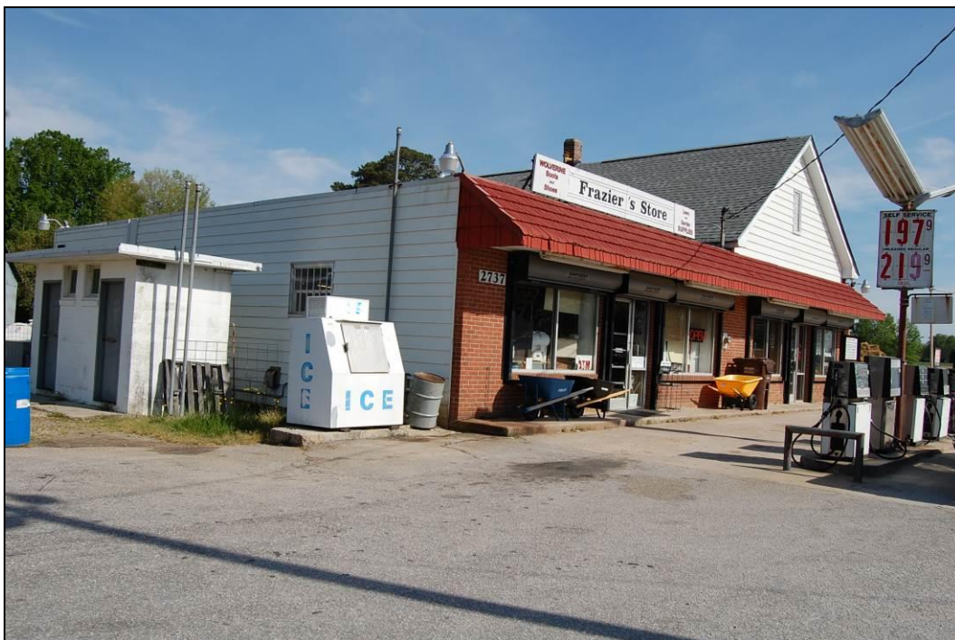
Figure 37. Southeast front and southwest side elevations of store; note freestanding bathroom building at far left
