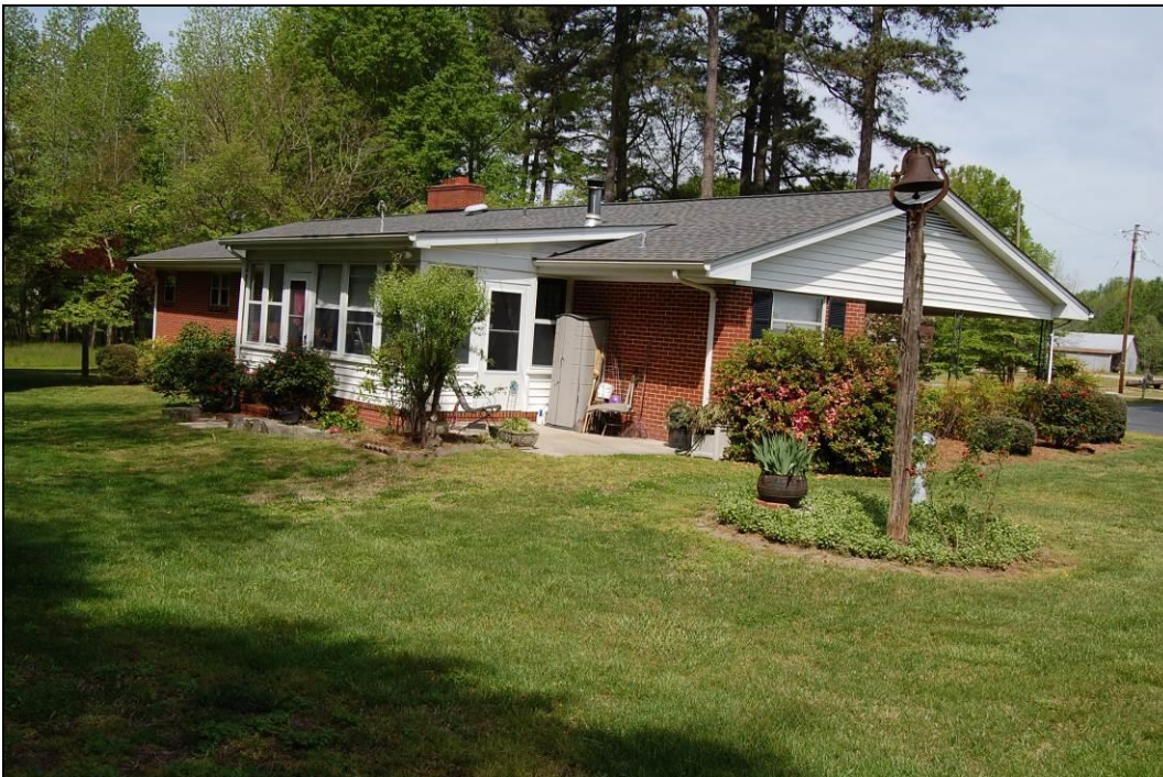
Figure 55. South rear and east side elevations of house
