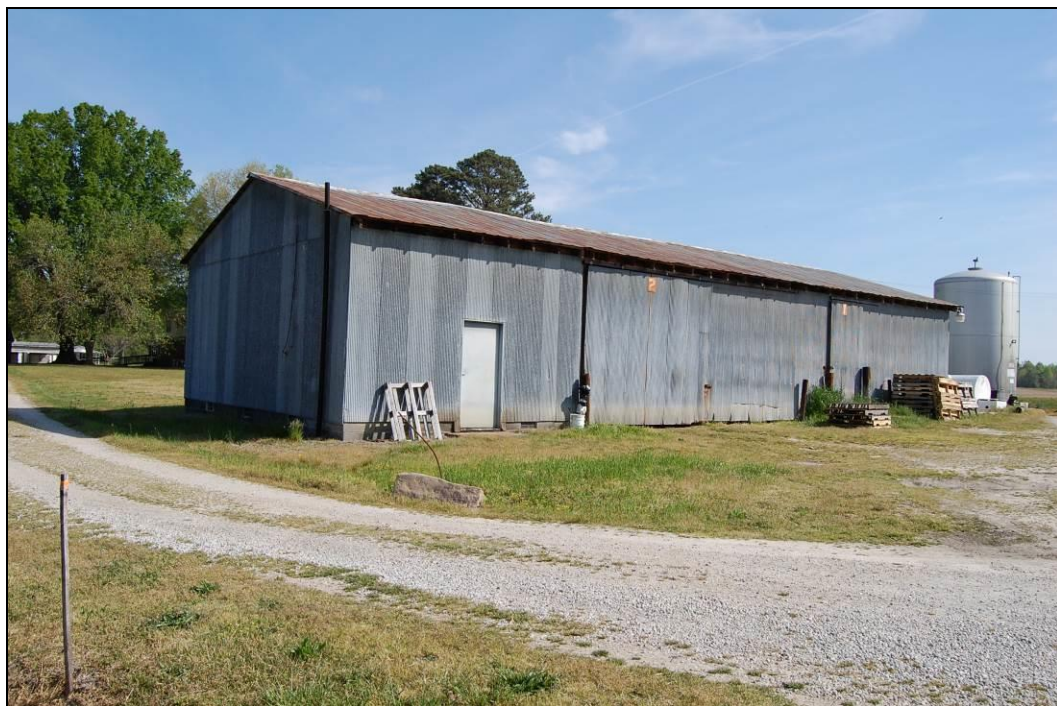
Figure 41. Looking northeast at storage building and fuel tank
