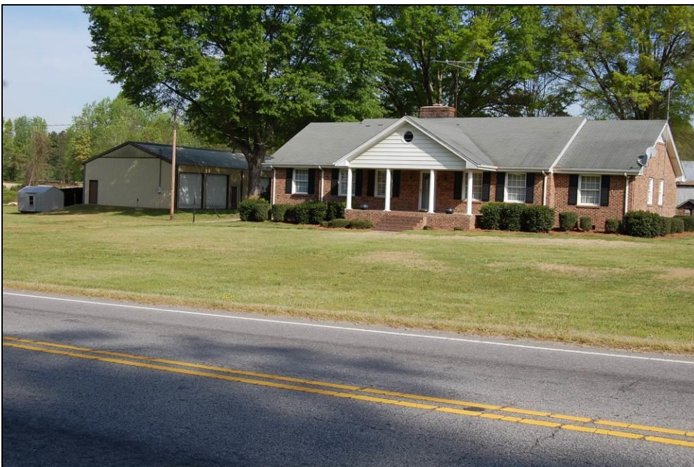
Figure 27. South front and east side elevations of house; garage at left
