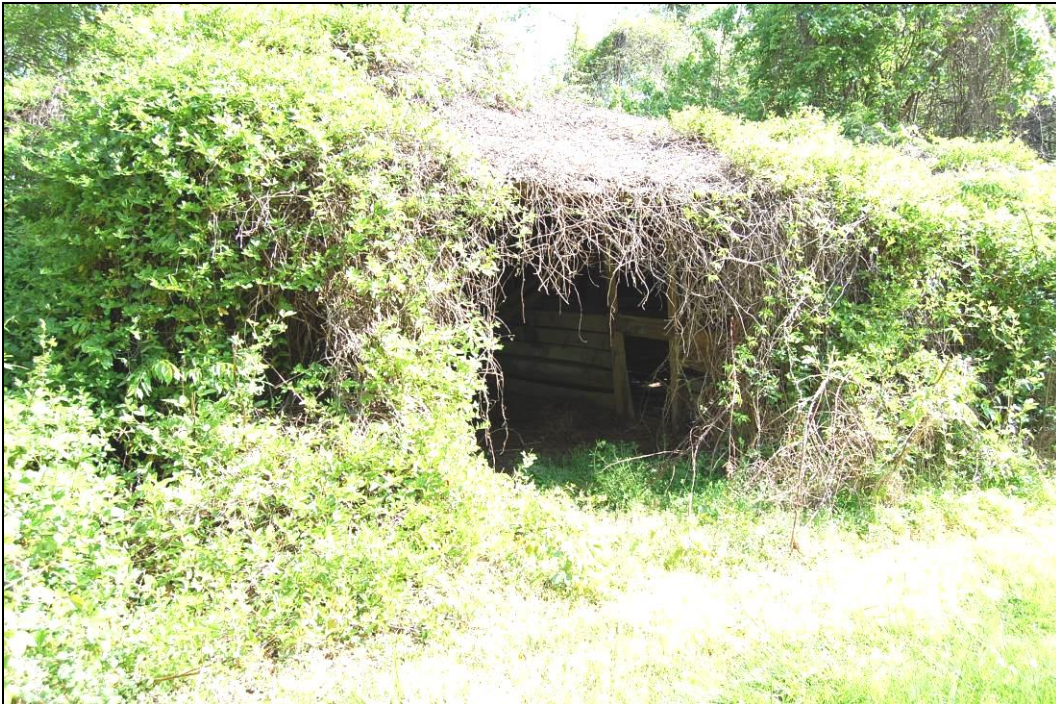
Figure 49. Looking northeast at shed engulfed by vines
