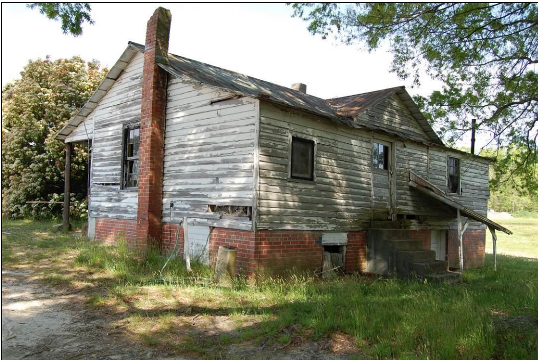
Figure 44. South side and east rear elevations of house
