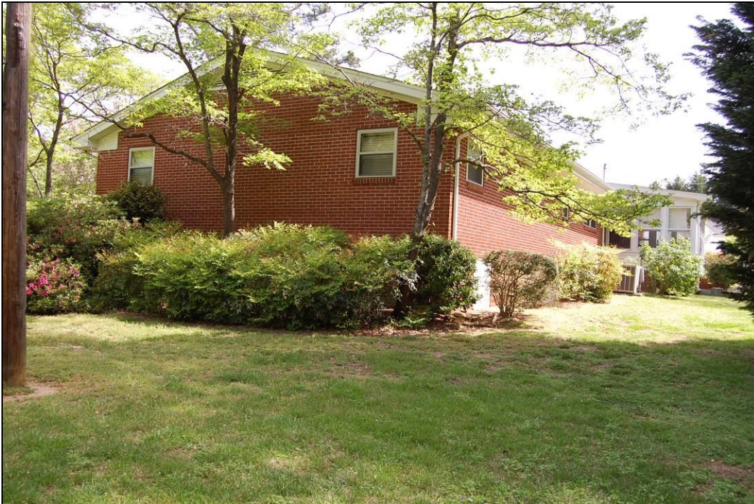
Figure 56. West side and south rear elevations of house
