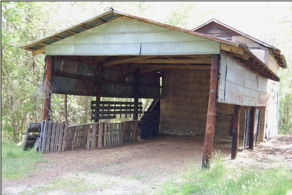
Figure 51. Looking northeast at shed and tobacco barn
