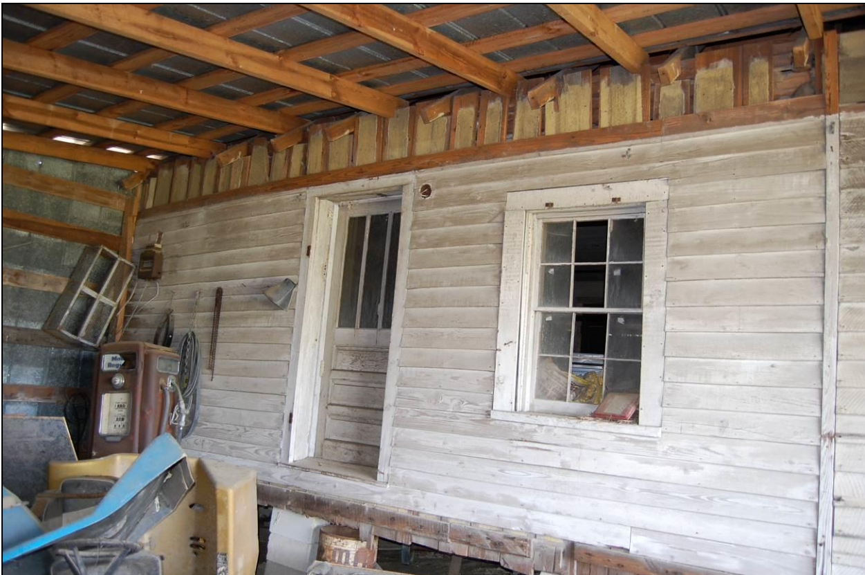
Figure 21. Former tenant house/outbuilding [7], looking northwest at south elevation of log section
