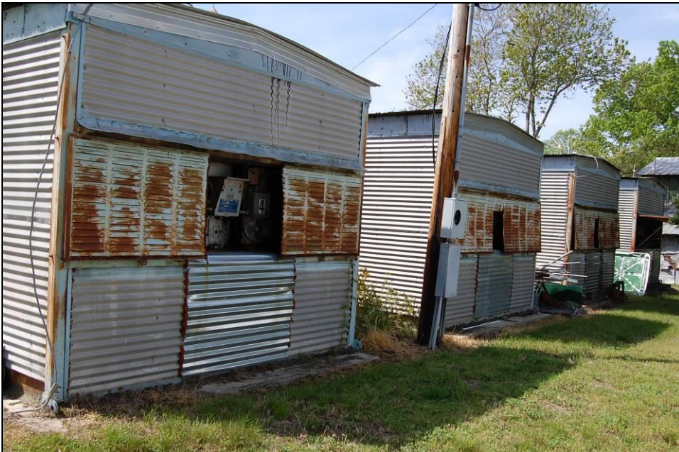
Figure 23. Bulk barns [8], looking south
