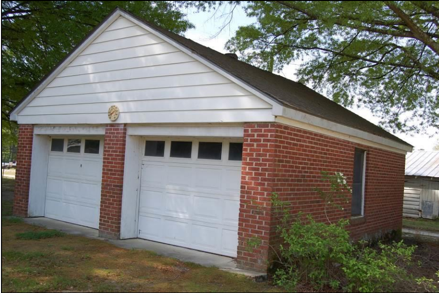
Figure 14. Garage [2], east front and north side elevations
