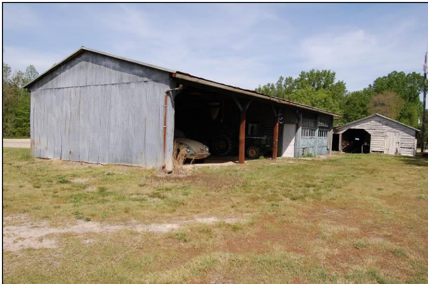
Figure 17. Tractor shed [5] at center and shed [4] at right, looking northwest
