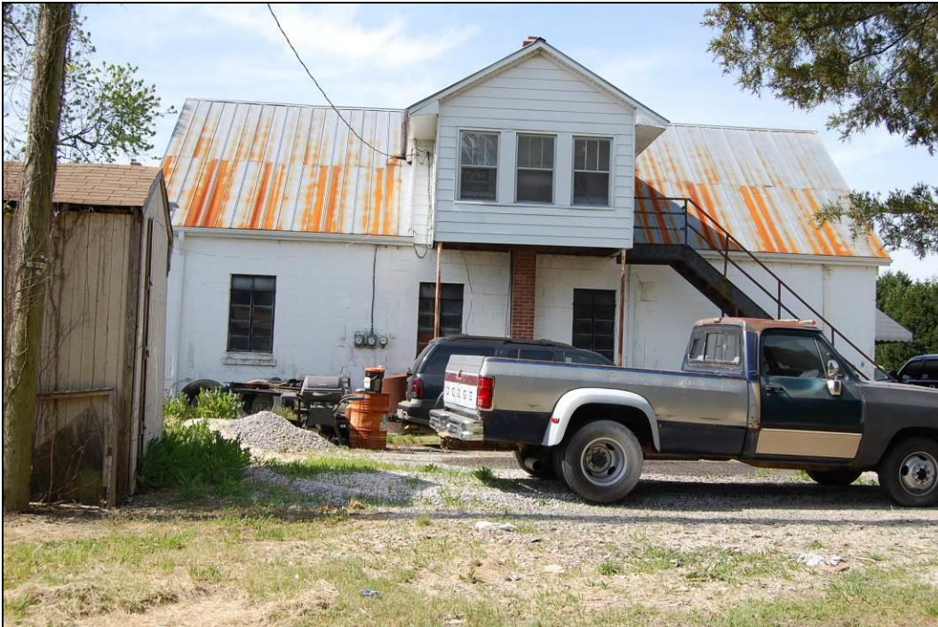
Figure 66. Northeast side elevation of garage; note modern frame shed at left
