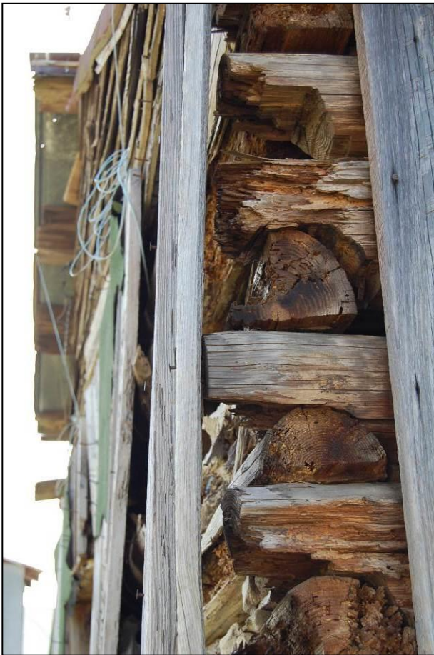
Figure 31. Detail of log construction at north gable end of store
