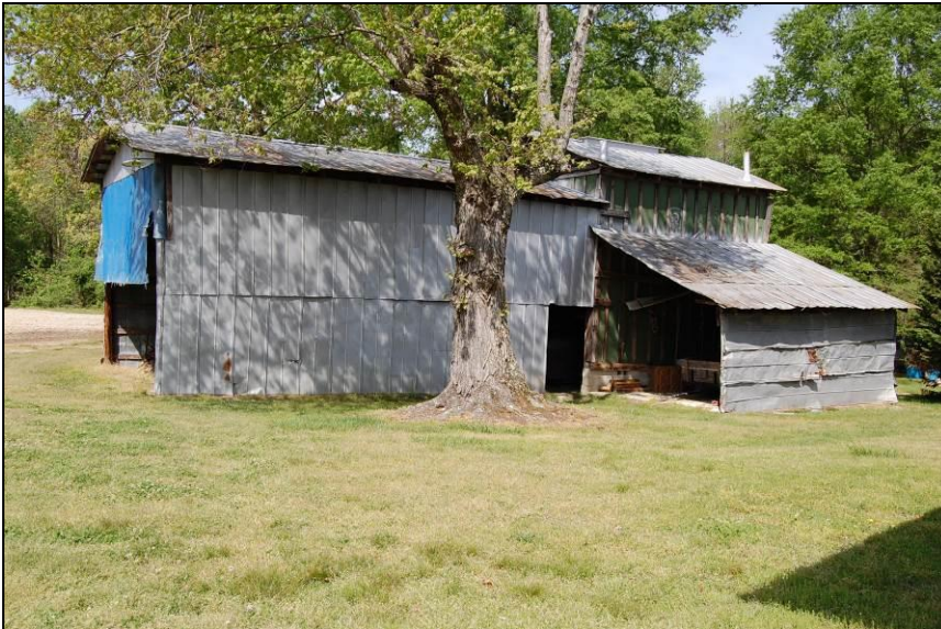
Figure 24. Tobacco barn and sheds [9], looking northwest
