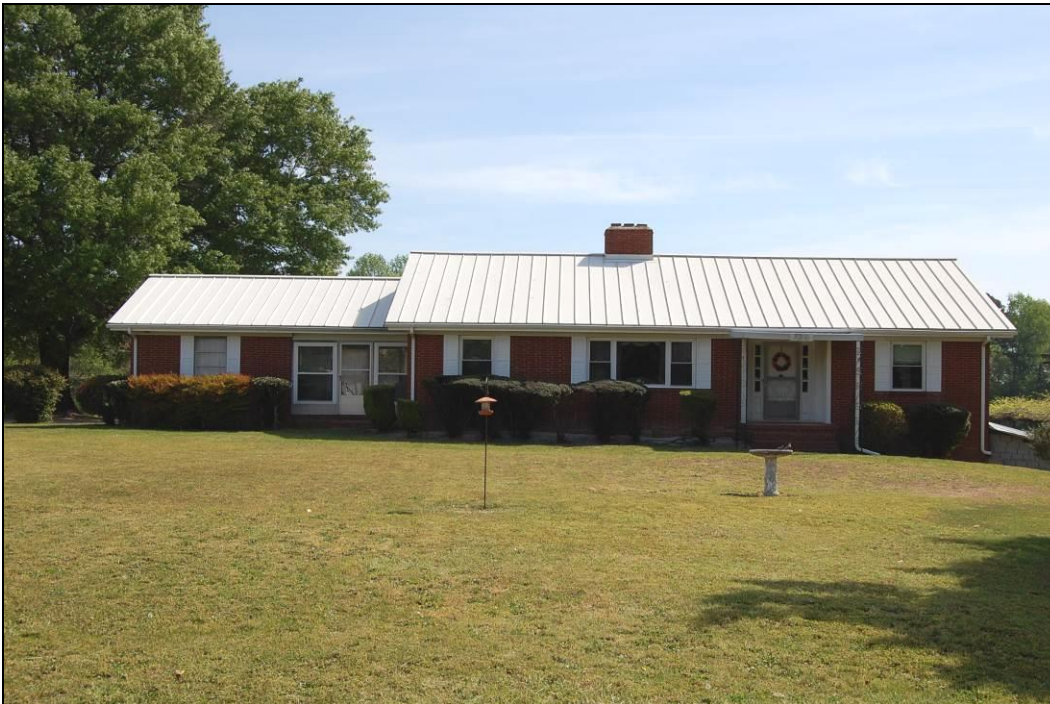
Figure 70. West front elevation of house
