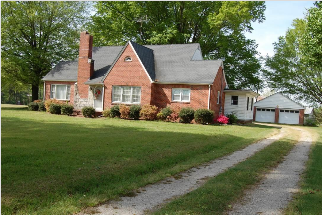
Figure 12. House, east front and north side elevations; garage [2] at right
