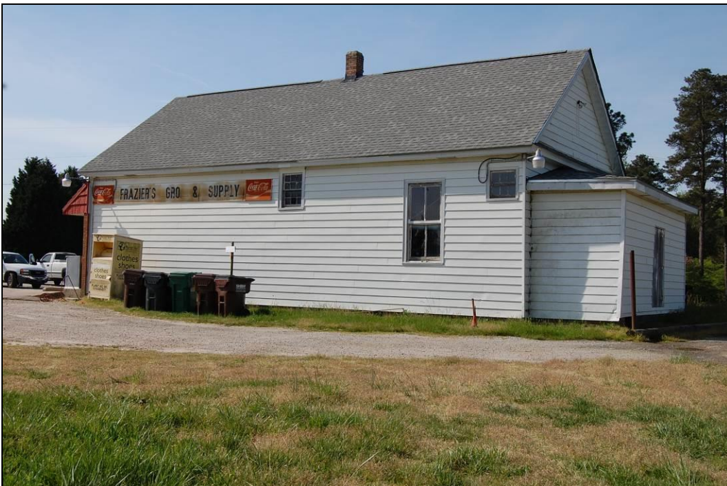
Figure 39. Northwest rear and northeast side elevation of store
