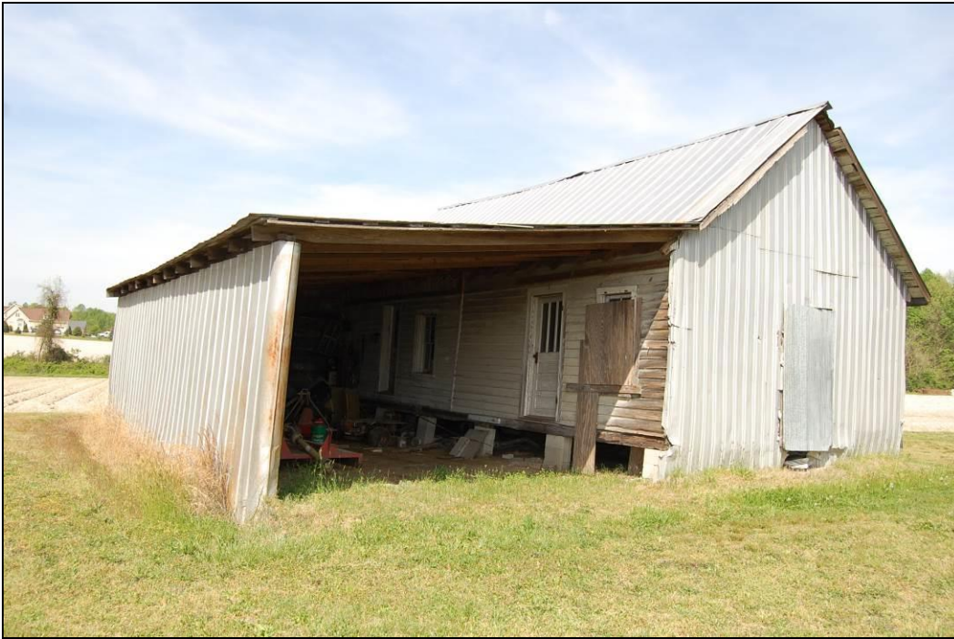
Figure 20. Former tenant house/outbuilding [7], looking northwest
