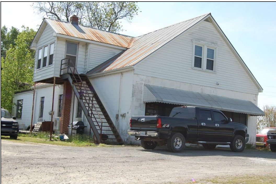
Figure 63. Northeast side and northwest front elevations of garage
